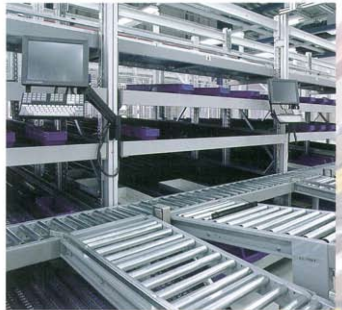
The SELECTAFLO solution, above, is fully integrated to the warehouse management system and will effortlessly handle up to 20,000 loads a day.
